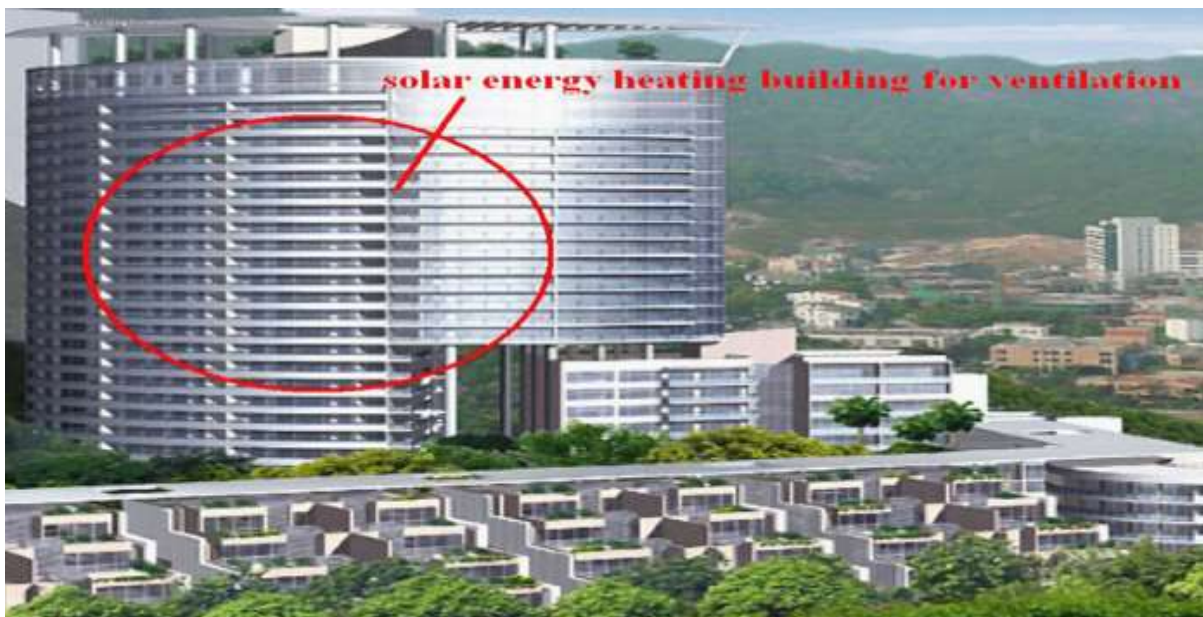
Fig. 3. Solar heating of building with trombe wall for natural ventilation(Li et al,2007).
